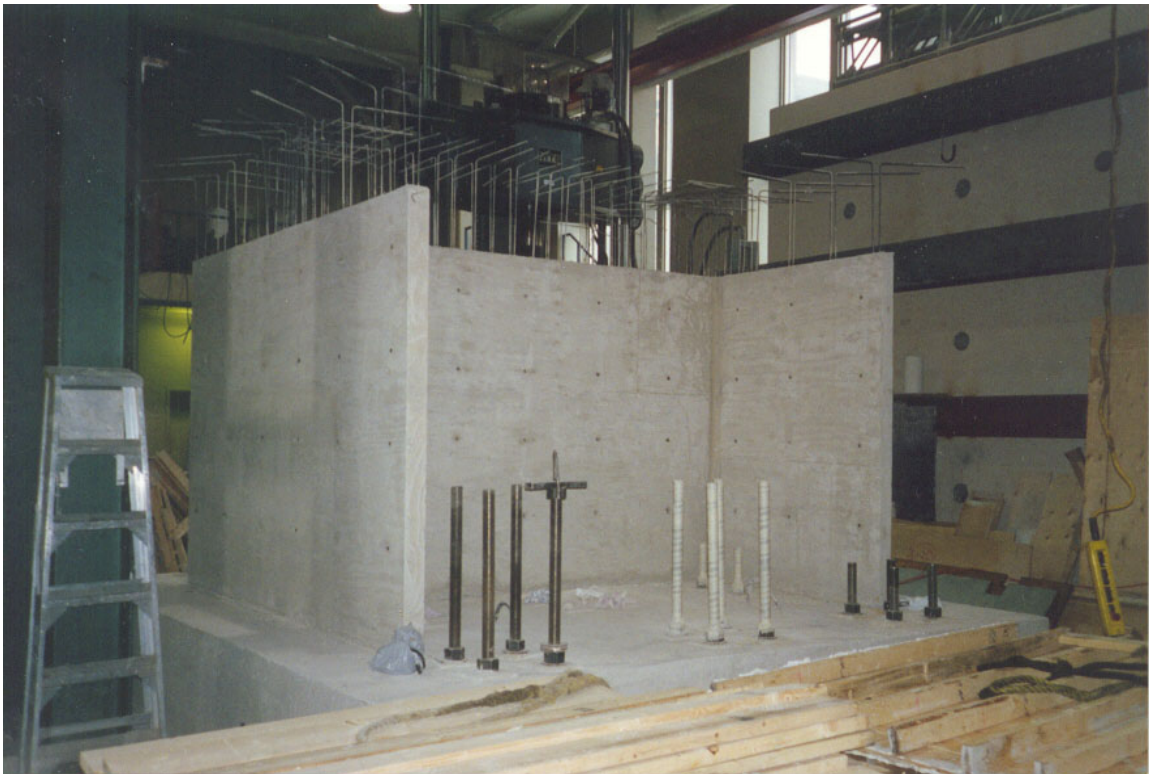
Figure 4.15 Walls After Casting
