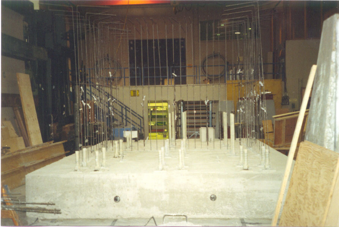
Figure 4.14 Base Slab After Casting
