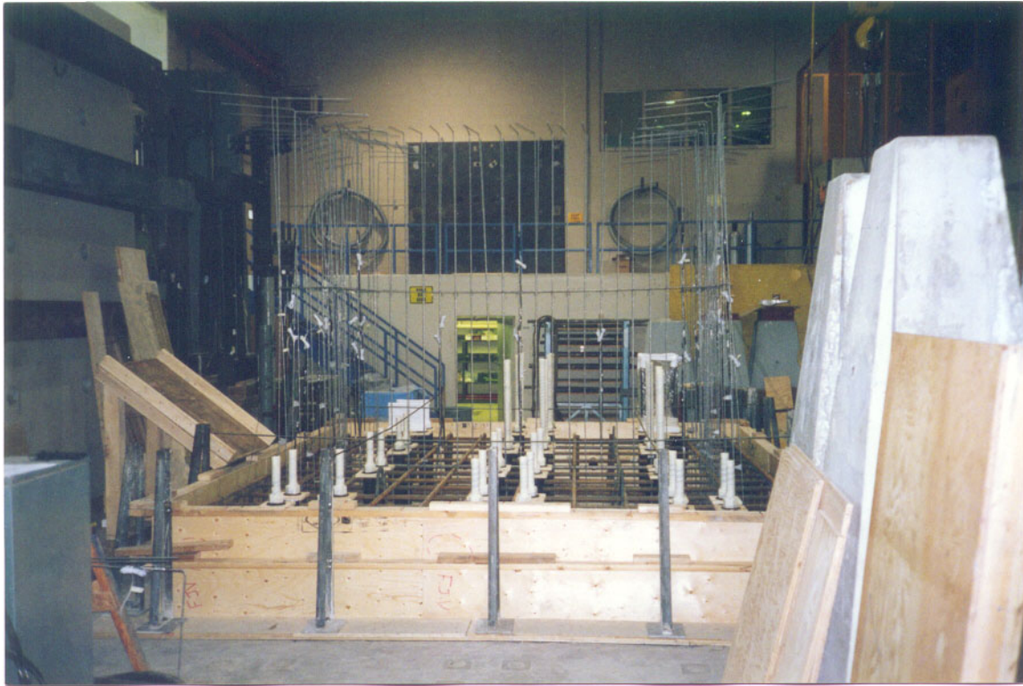
Figure 4.13 Base Slab Prior to Casting
